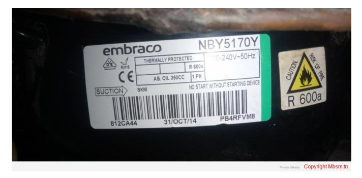
File Pdf: NBY5170Y, Compressor, 1/4 HP, 1ph 220-240V/50Hz, R600a, 15kg, High Back Pressure, HBP, Commercial Refrigeration, Embraco
